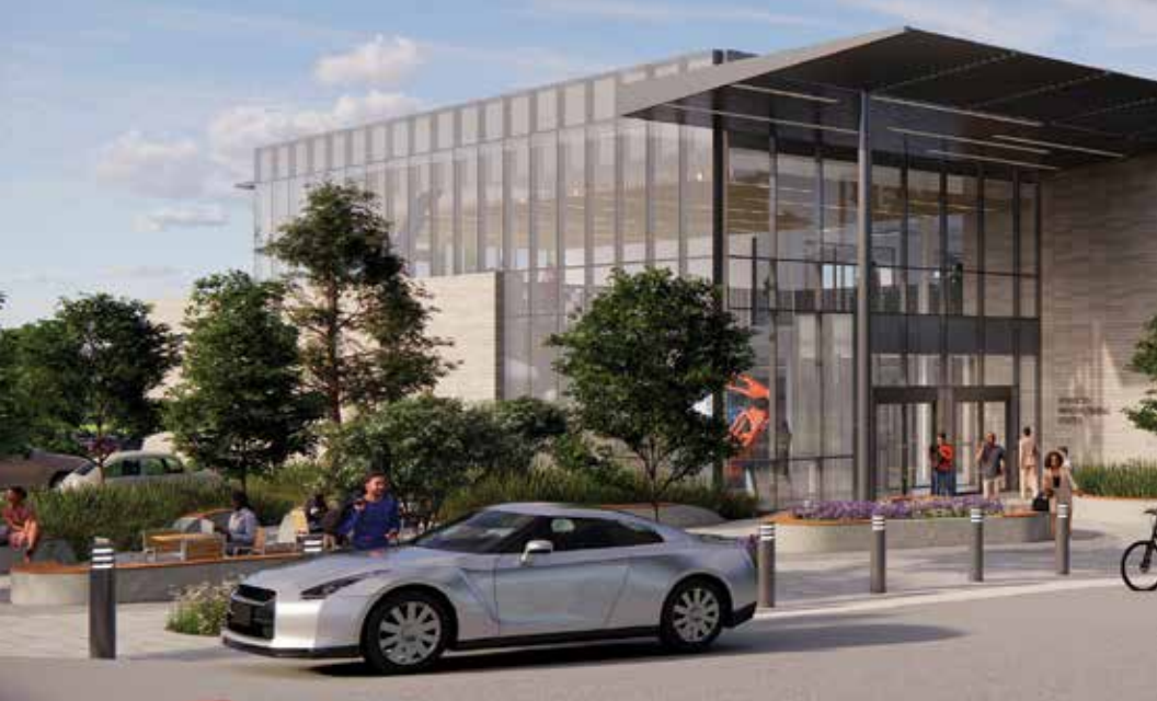
Future home of the Boeing Pre-Employment Training Program at the new Center for Advanced Manufacturing at the Florissant Valley Campus (Photos courtesy of STLCC)
